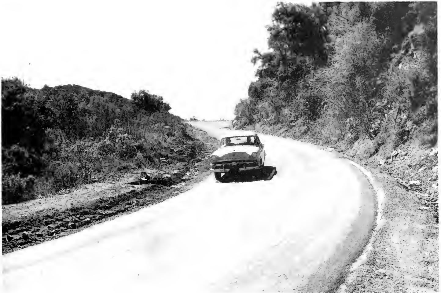
Type of curve which will be eliminated on San Marcos Pass Highway. This view is looking north.
